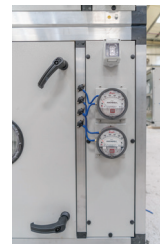
Fig 16: Magnehelic Gauge
