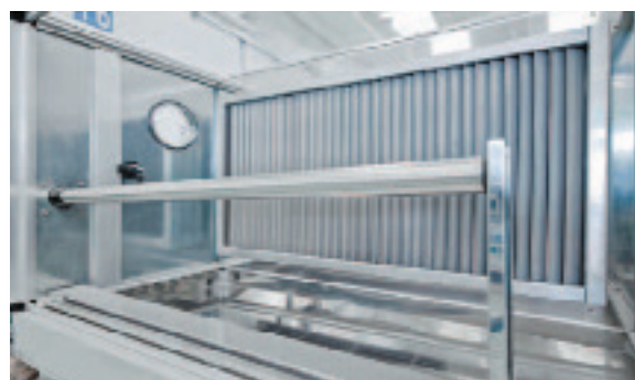
Fig 37: Steam Humidifier
