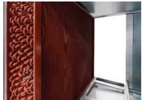
Fig 20: Coils with Herasite Coating
